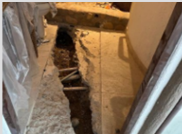
Major repairs to the A.C. condensation line and electrical in the Junior Bedroom. Some VERY serious work (major "surgery" involved to the walls and floor! Similar repairs were also done in Villas 3 and 5.
