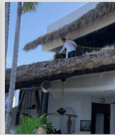
Palapas were treated with fire retardant.
