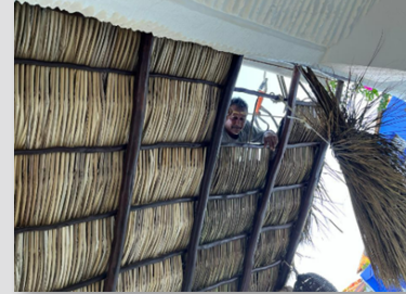
Palapa repairs. (Yes, done from outside, on top!)
