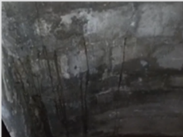
A leak was found in one of the elevator shafts and repaired.
