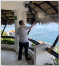
Palapas were treated with fire retardant.
