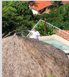
Palapas were treated with fire retardant.
