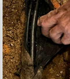
Extensive work required to repair the AC condensate lines in the Junior Bedroom. Wall and floor had to be dug-up! This work will be required in Villas 2, 7, 8 & 9 next September.
