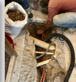
Extensive work required to repair the AC condensate lines in the Junior Bedroom. Wall and floor had to be dug-up! This work will be required in Villas 2, 7, 8 & 9 next September.
