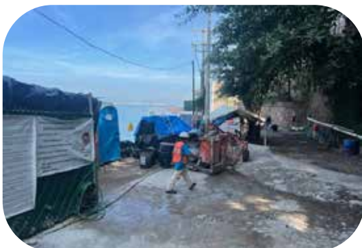
At Calle Santa Barbara looking north
